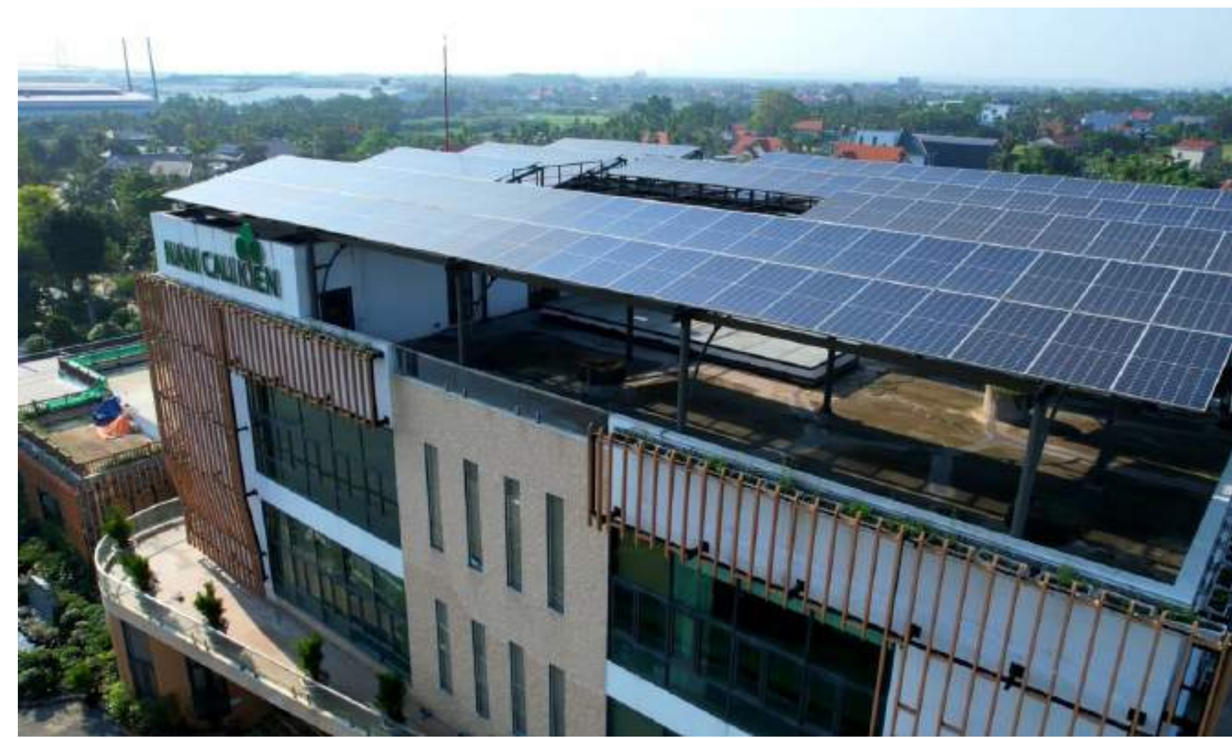
Solar power has been implemented
