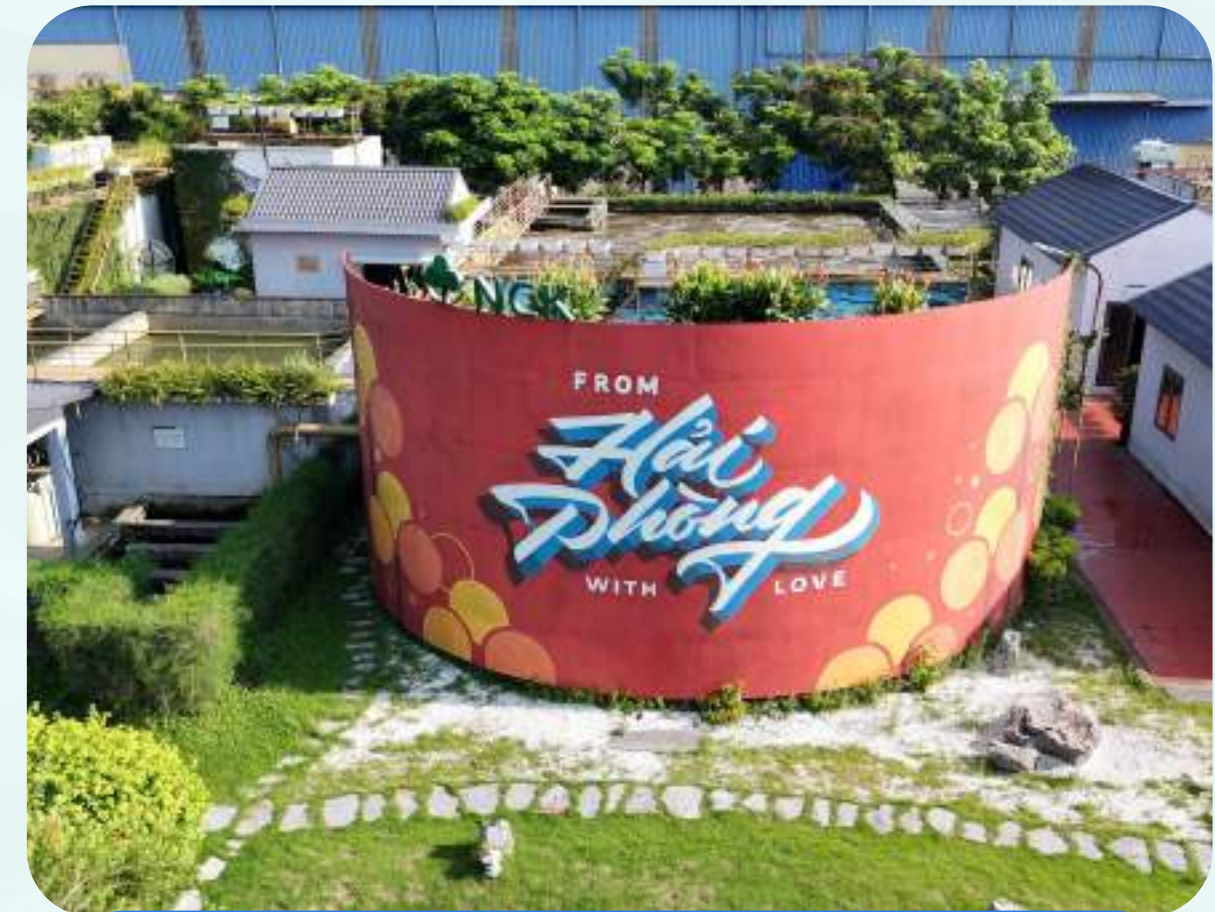
Japanese garden wastewater treatment plant
